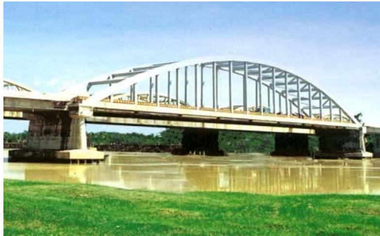
Gambar 6. Jembatan Cindaga, Jawa tengah, 1979 double Plane Arch Concrete Bridge, Bentang 90 meter.
