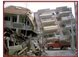
Figure 2: Earthquake damage of a building
