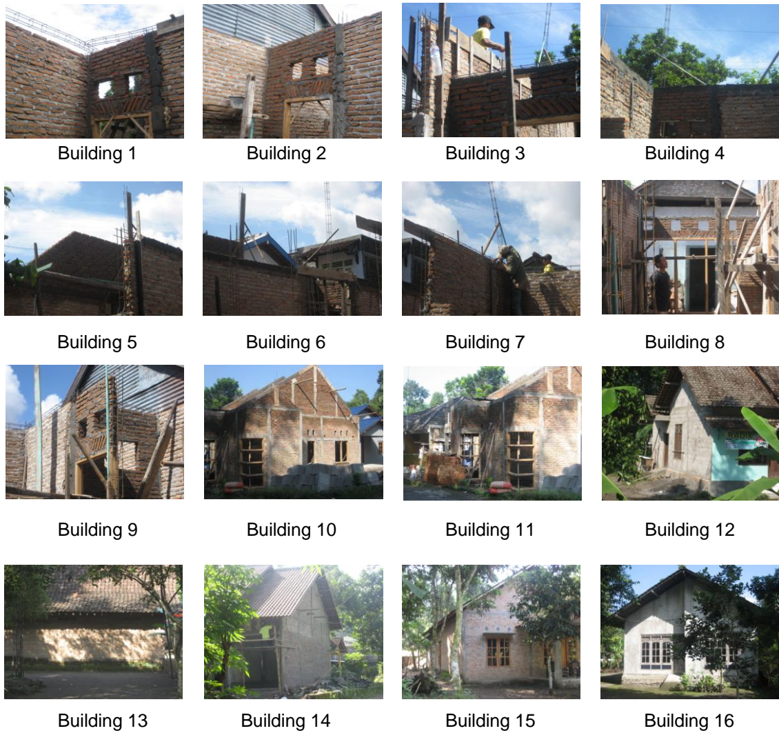
Figure 4. A set of building photographs
