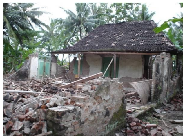
Figure 6. Comparison between still standing combined structure and purely brick wall house
