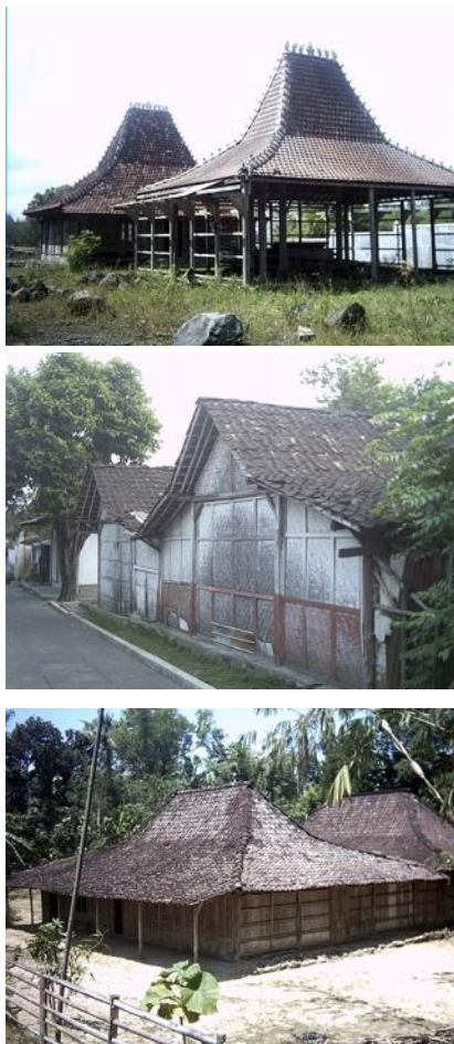
Figure 1. Original Javanese Joglo, Limasan, and Kampung types with clay roof tile and wooden materials from hard wood to bamboos
