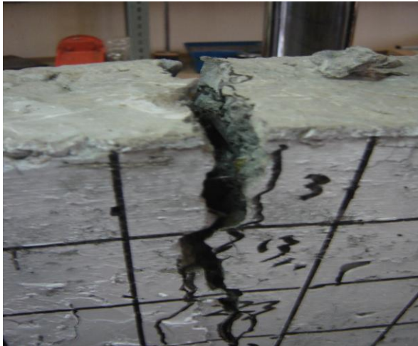
Figure 6. Crack at middle span of beam specimens at ultimate stage (Susilorini, 2009b)
