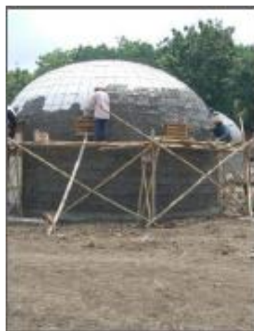
Figure 20. Casting concrete monolith. (Source: DFTW, 2008)
