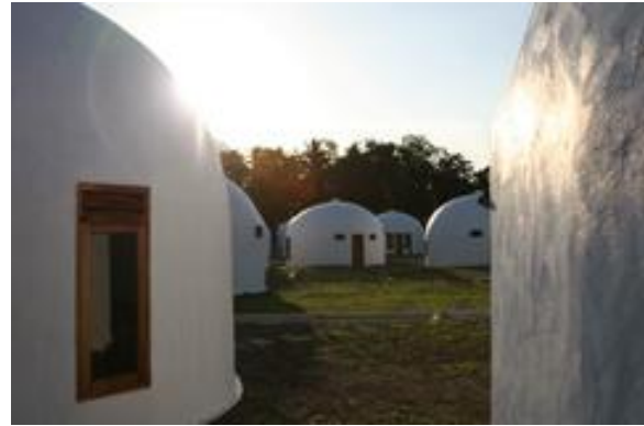
Gambar 18. The non-orientation causes the dome can not minimize espousing to the sun during the dry season (Source image: Eeghout, 2008)
