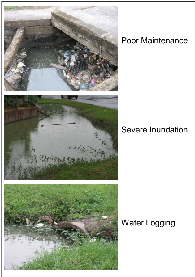
Figure 3 Current condition of existing drainage and contributing drainage system
