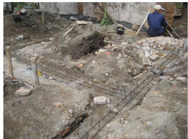
Figure 2. Building reinforcing steel bars
