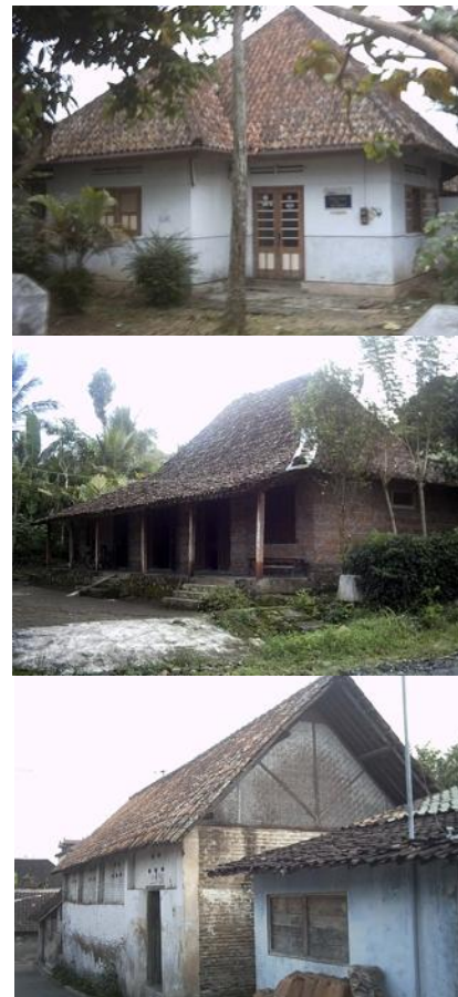
Figure 2. Old Culture houses; Dutch high pyramidal roof, Javanese Limasan, Javanese Kampung with masonry bearing wall structure
