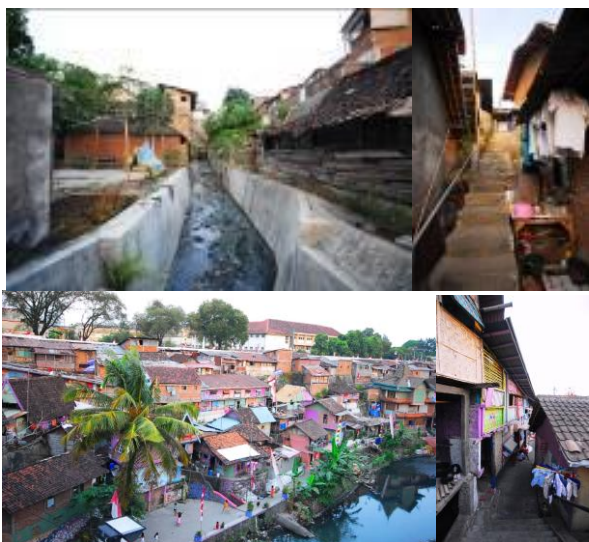
Figure 3 Typical condition of high density residential (The example is taken from residential kampung along Code River in Jogjakarta)
