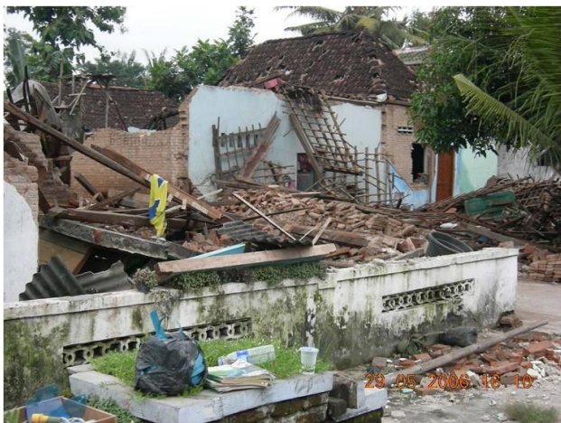
Figure 3. Javanese old culture houses collapsed
