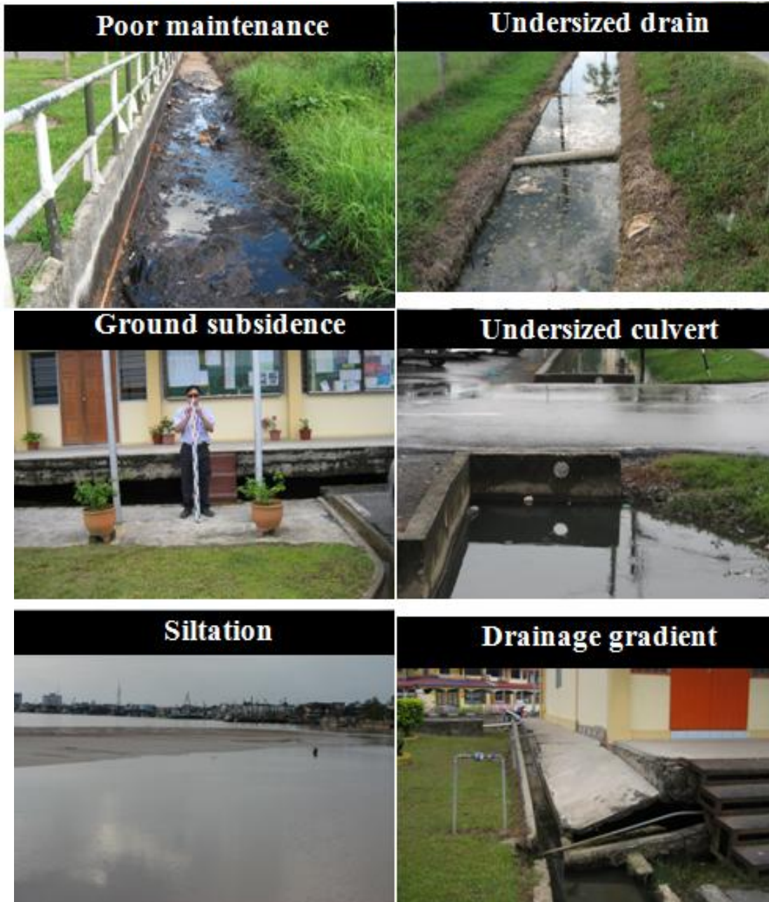
Figure 8 Current situations that causes flood to Sibul Town
