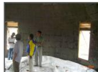
Figure 21. When finished casting (Source: DFTW, 2008)
