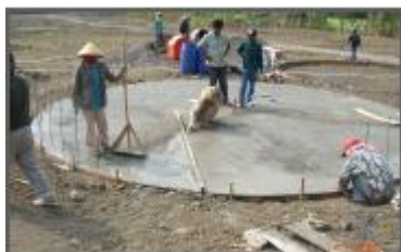
Figure 19. Casting molds and preparation of concrete floors balloon (Source: DFTW, 2008)
