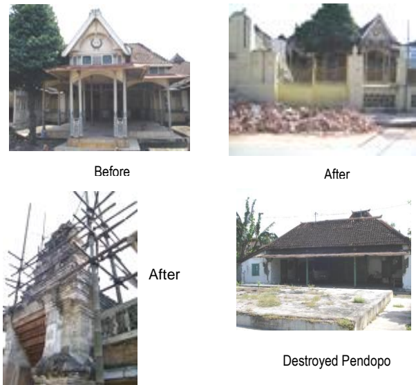
Figure 6. Damage in Kotagede after earthquake Reference: Oktaviyani (2008)
