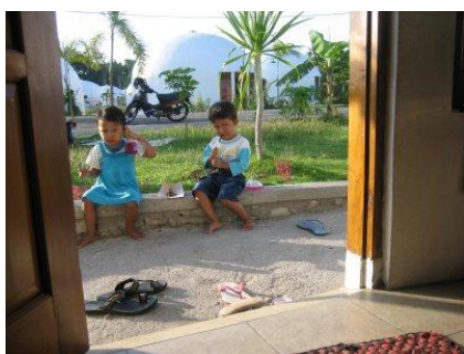
Figure 22. Solar radiation in the absence of direct entry porch as shading. In addition to the entry of radiation will cause the heat of the scorching sun, this condition will also allow the rain water come into the room when the rain came.
