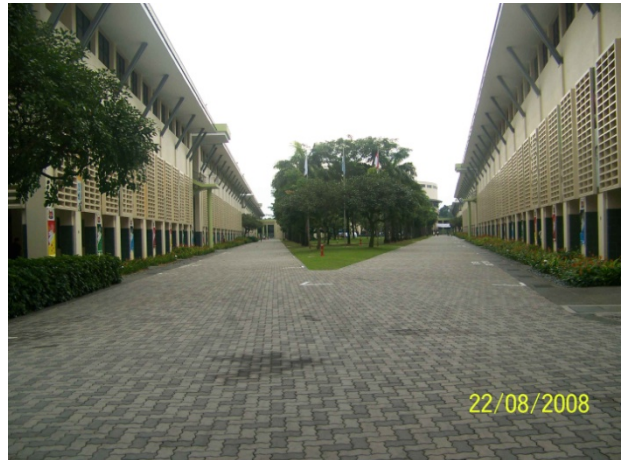
NIE Building Complex
